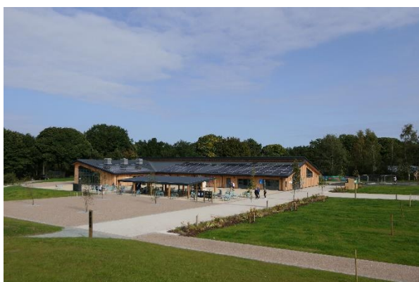
Figure 4: The completed Delamere site
