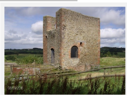
Above: The old engine house for Ladywell Lead mine. (SAM) but not FC
