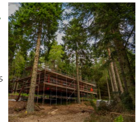
Cabin being erected within scaffolding
