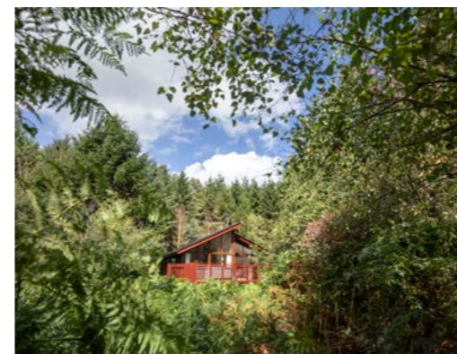
No gutters so rainwater drains into the forest floor naturally
