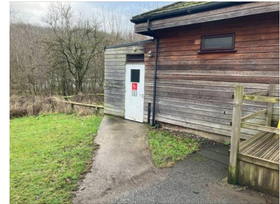
Step free path to accessible toilet on left side at rear of toilet block
