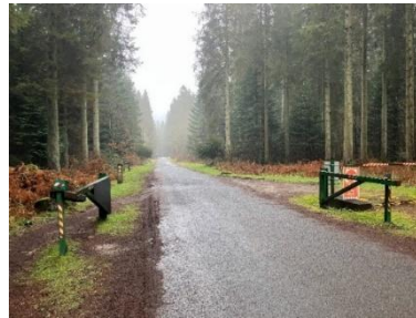
The Grove Barrier - Open
