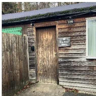
Pine room entrance, showing small, ramped access and black lock box
