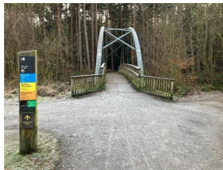
First Bridge Crossing
