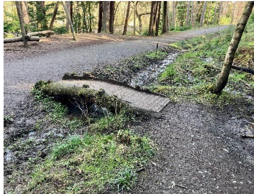
Small bridge from main path to the play area
