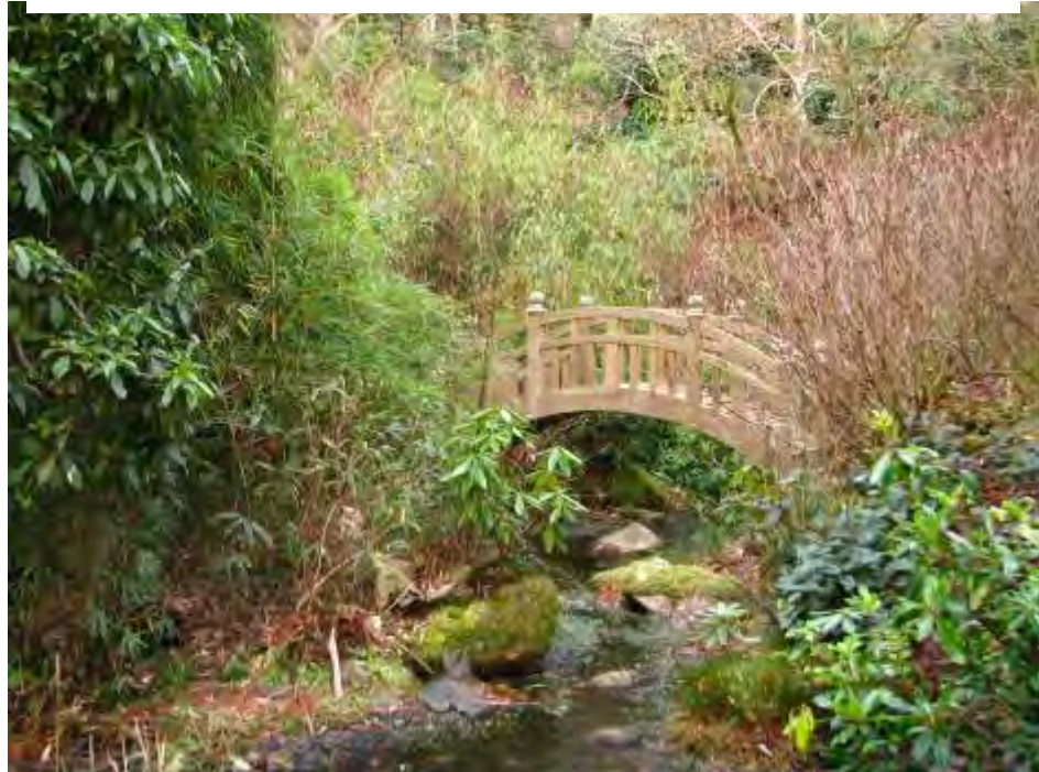
With funding from Eskdale Parish Council three bridges were constructed and erected by a local joiner to restore routes across the water feature.
