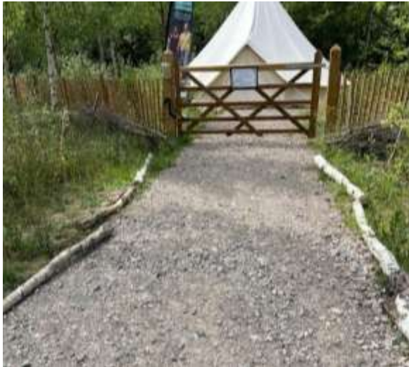
The path that leads to the entrance to the Den is wide, with loose stones. There is a wooden gate at the entrance.
