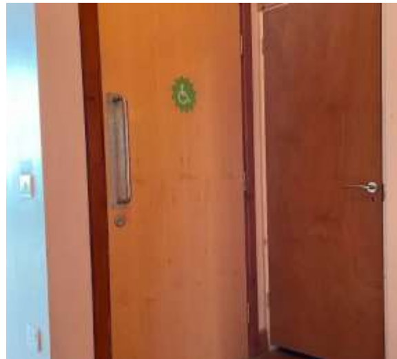
There is one accessible toilet inside the toilet block, this does not require a RADAR key to open.
