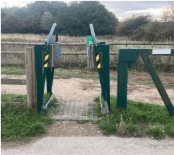
Motorbike deterrent gate at the New Fields Road entrance.
