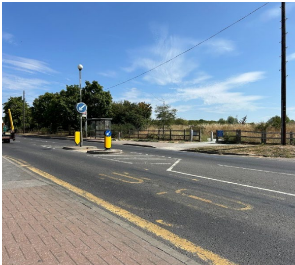
The pedestrian and cycle path entrance from Rainham Road via a pedestrian crossing.
