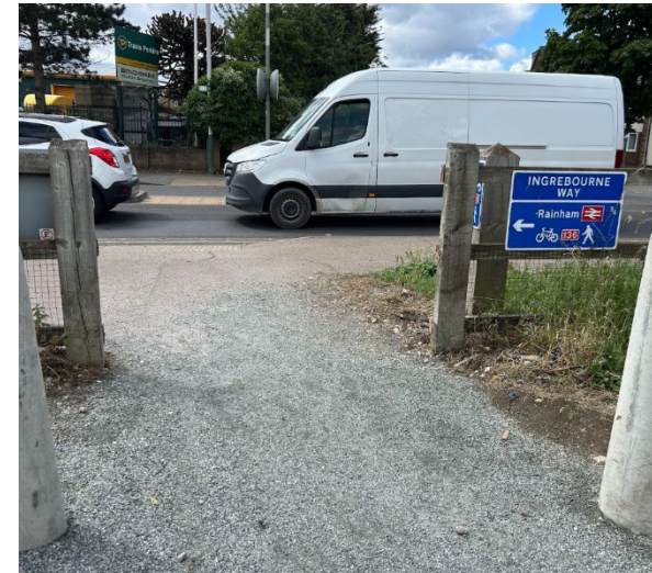
Access gap into Ingrebourne Hill from Rainham road which is more than 1m wide.
