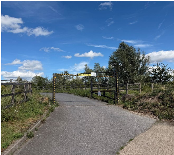
The main vehicle entrance on Rainham Road has a 2m high vehicle barrier.
