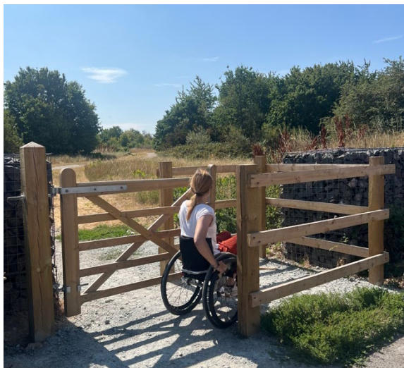
Wheelchair accessible kissing gate provided on the Conifer Loop pedestrian entrance via South End Road. This may not be large enough for some mobility scooters to turn.
