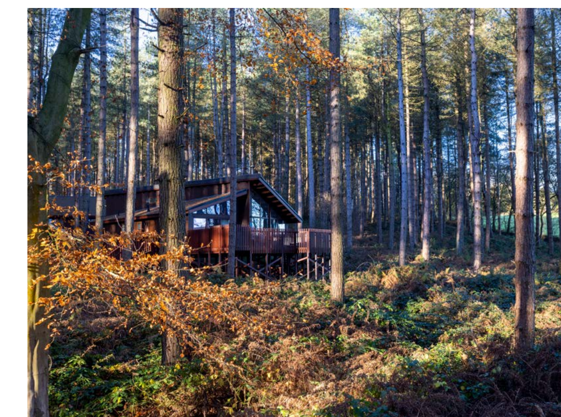
Example of new cabins created in Delamere Forest in 2021
