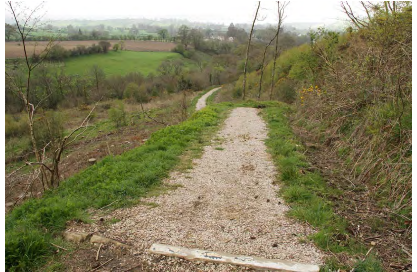
The improved section of the Cumbria Way.
