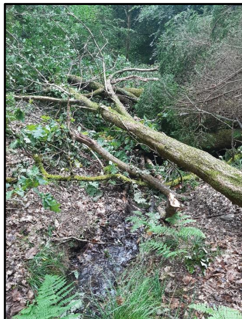
Figure 20 (left and far left) Trees have been felled into Ropehouse Ditch to slow the flow of water
