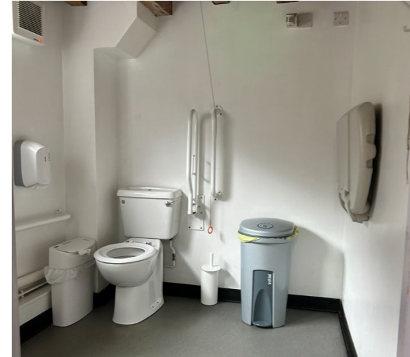
The accessible toilet has a right-hand transfer. The toilet cubicle is a standard size, with grab rails fitted and an emergency pull cord.
