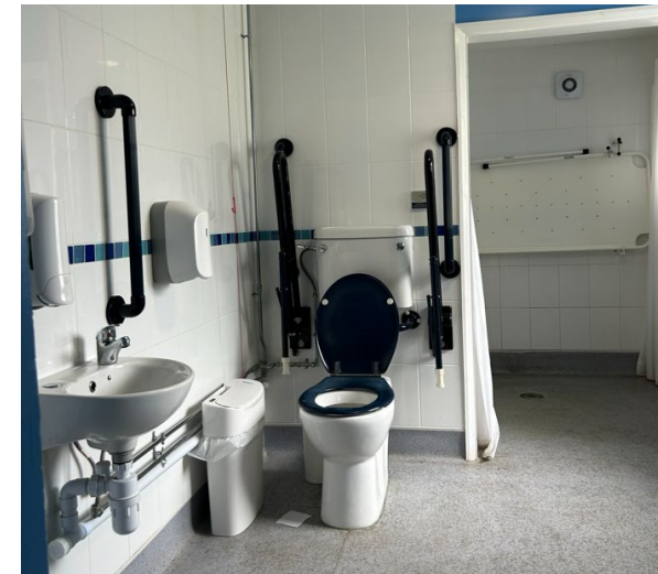
The adapted cubicle is larger than a standard accessible toilet, it is fitted with drop-down grab rails on either side of the toilet. There is an adult changing bench at the back of the room.
