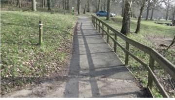
Access to the lodge from Area 1 can be gained using a DDA compliant (Equality Act 2010) tarmac ramp, which has a handrail to one side (halfway)
